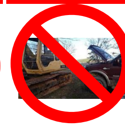
Charging batteries via jump leads attached between two items of plant
