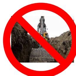
The use of mechanical equipment within utility exclusion zones
