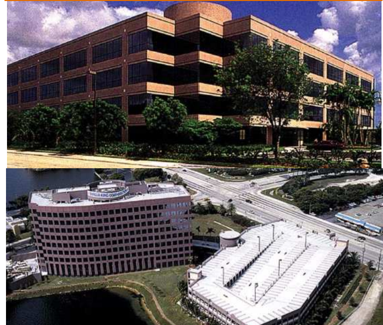
8 Waterford Office Projects
