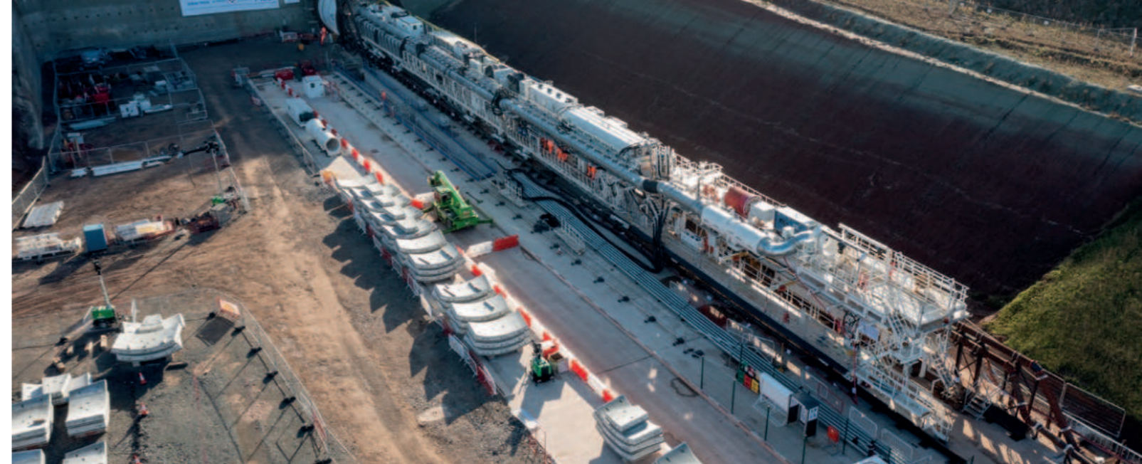
HS2 Main Civil Engineering Works
