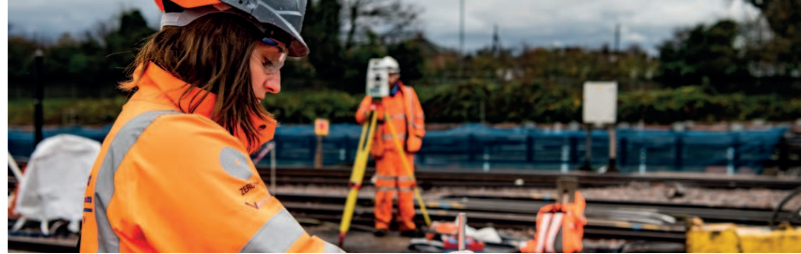
London Underground Track Renewals
