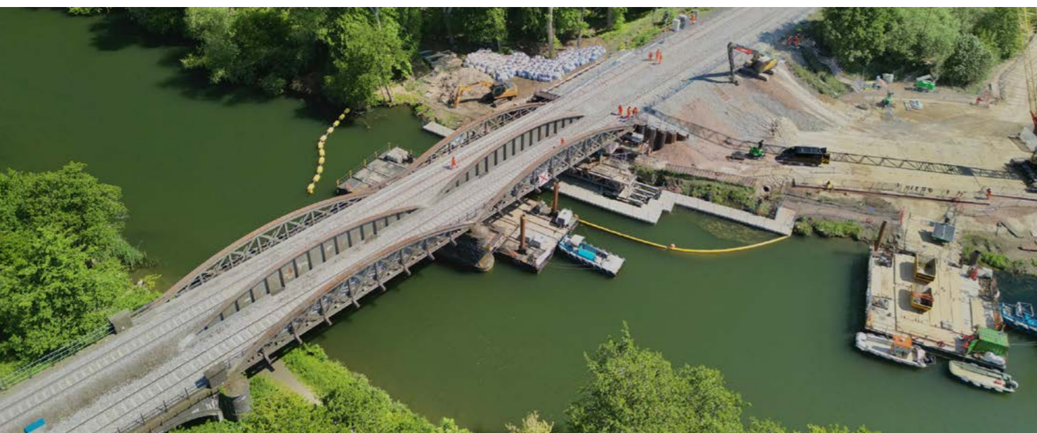
Nuneham Viaduct restoration, Oxfordshire
