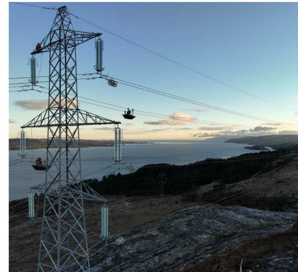
Port Ann to Crossaig Overhead Line Works
