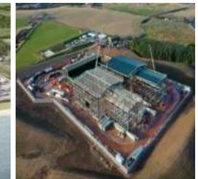
Offshore wind connection and base construction
