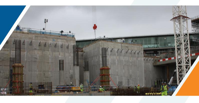
Diaphragm walls are underground structural elements commonly used as retention systems and permanent foundation walls. They can also be used as groundwater barriers.
