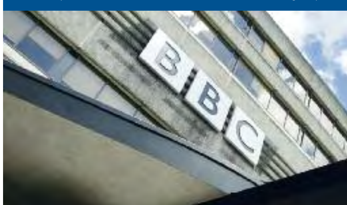
Balfour Beatty WorkPlace's contract with the BBC was extended during the year.
