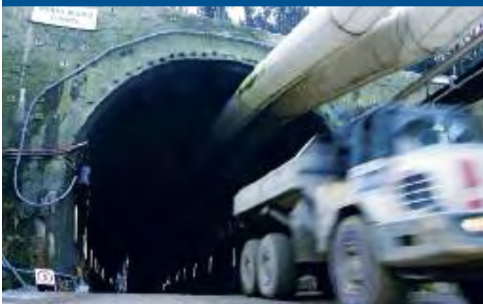
The A3 Hindhead improvement scheme made good progress.
