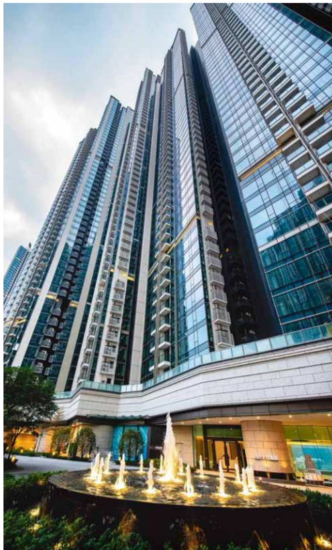
LEFT Lohas Park Package 9, development of three 54-56 storey residential towers for Wheelock and Company Limited, Hong Kong.
