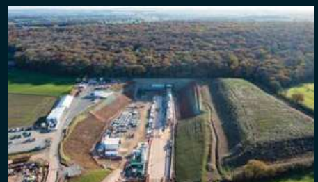
HS2 high-speed railway line, UK
