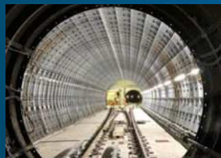
UK: London Underground Piccadilly line upgrade.
