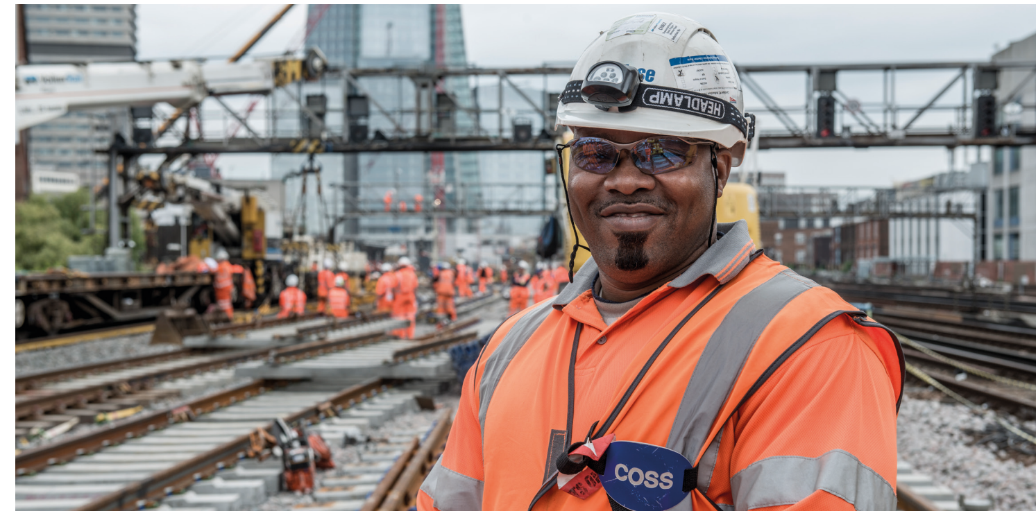
London Bridge station
