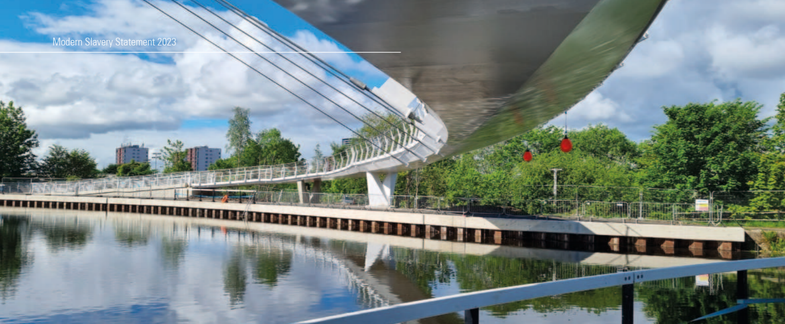
Stockingfield Bridge, Glasgow
