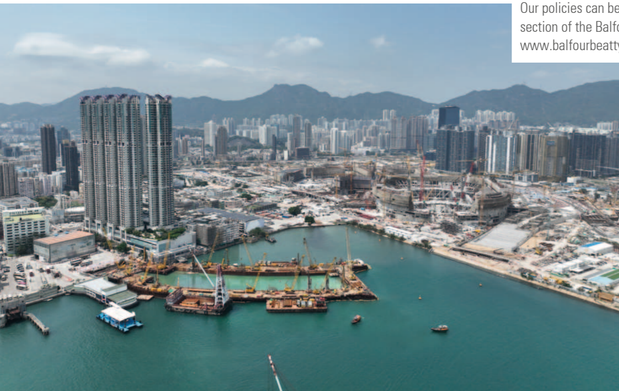
Central Kowloon Route - Kai Tak West Section, Hong Kong
