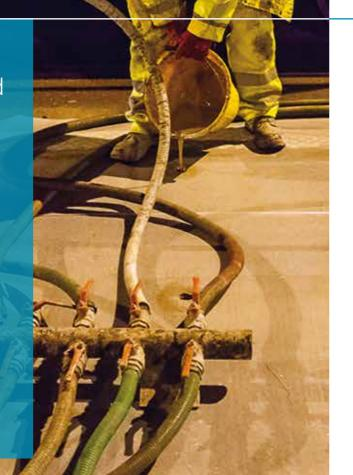
Concrete pavements, with or without a flexible overlay, are an important part of the UK road network. Voids can occur underneath these slabs that require specialist maintenance to enhance the life and integrity of the pavement and minimise the cost and disruption of replacing the carriageway.
