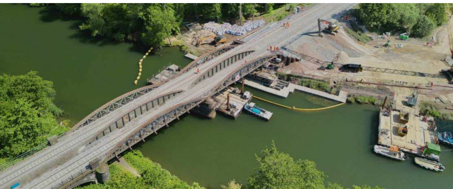
Nuneham Viaduct restoration, Oxfordshire
