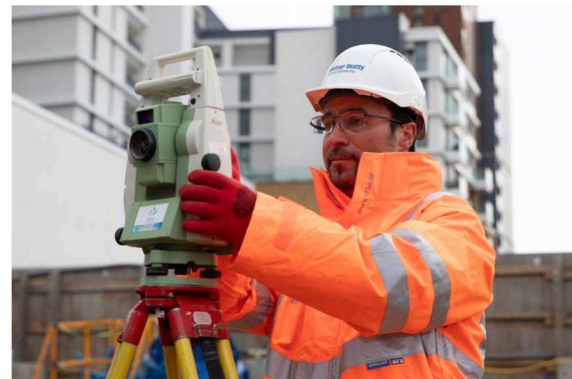
Northern Line Extension scheme, Nine Elms
