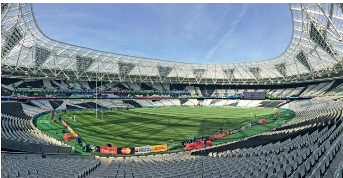
We're redeveloping and reconfiguring the Olympic Stadium into a 60,000 seat arena to host football, athletics and concerts.
