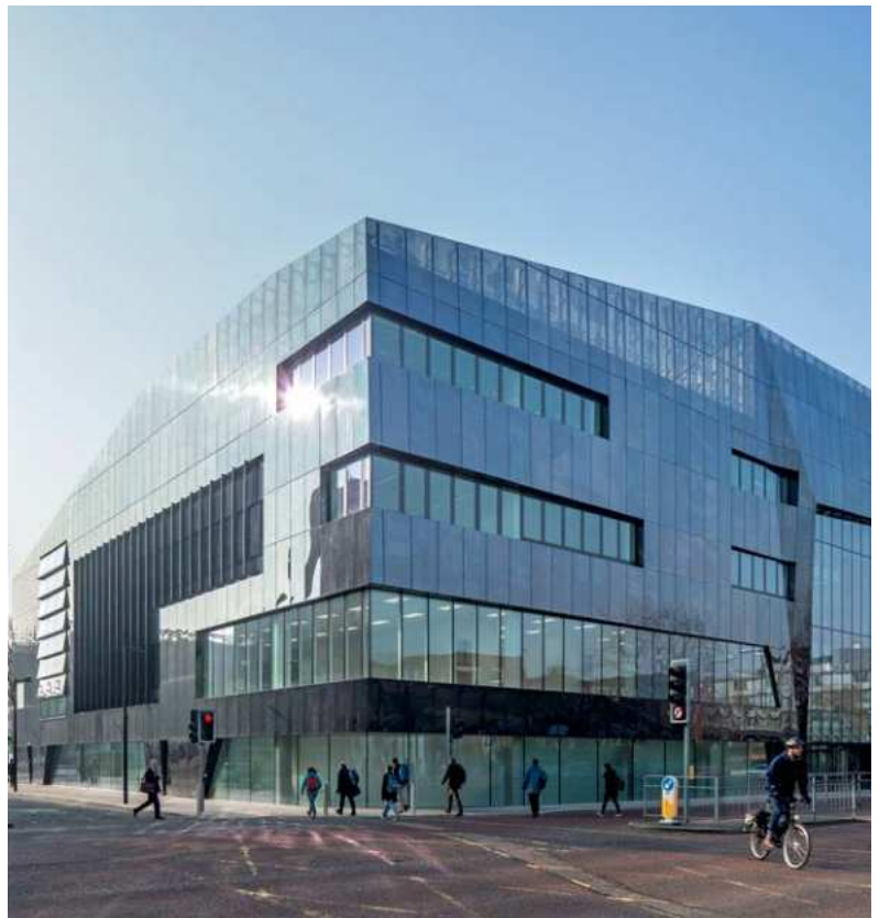
We delivered mechanical, electrical and process services for the leading edge facility that will carry out detailed research into Graphene.
