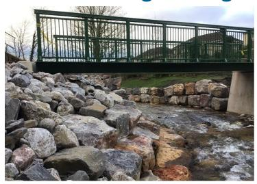
In November, a major milestone was reached on our project in Tyn-y-bryn with the arrival and installation of the brand-new footbridge. A section of the A4119 was temporarily closed overnight on 17 November to allow a 120-tonne crane to lift into position the new 11-meter footbridge.
