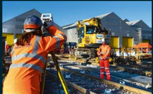
ABOVE UK: Ealing Common Depot track renewal, Transport for London
