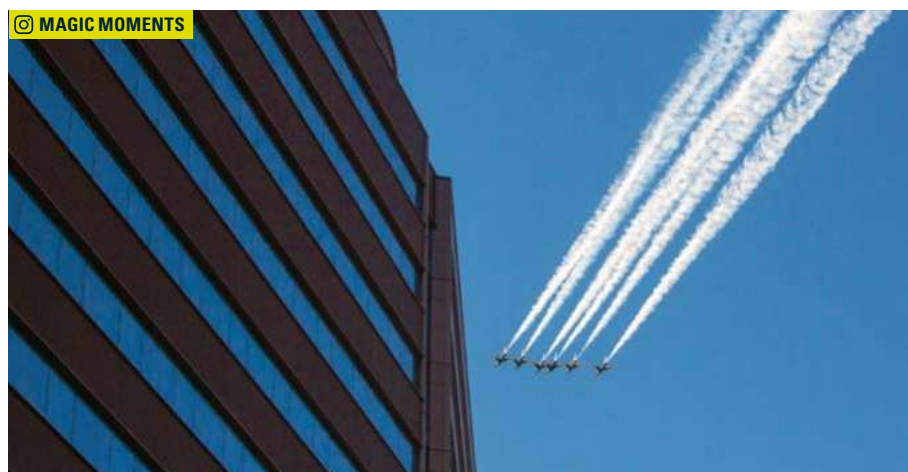
US: Thunderbird flyover over the Pavilion Penn Medicine project. Photo credit: Joseph Ebert
