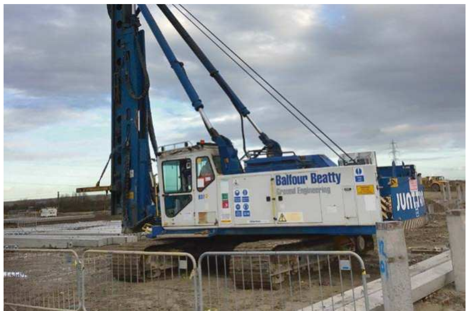
ABOVE First EU Stage V equivalent retrofit project on a Junttan piling rig
