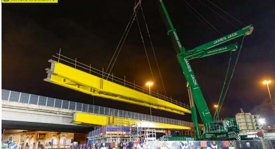
UK: Regent Street bridge lift, Leeds City Council. Photo credit: Catherine Morgan
