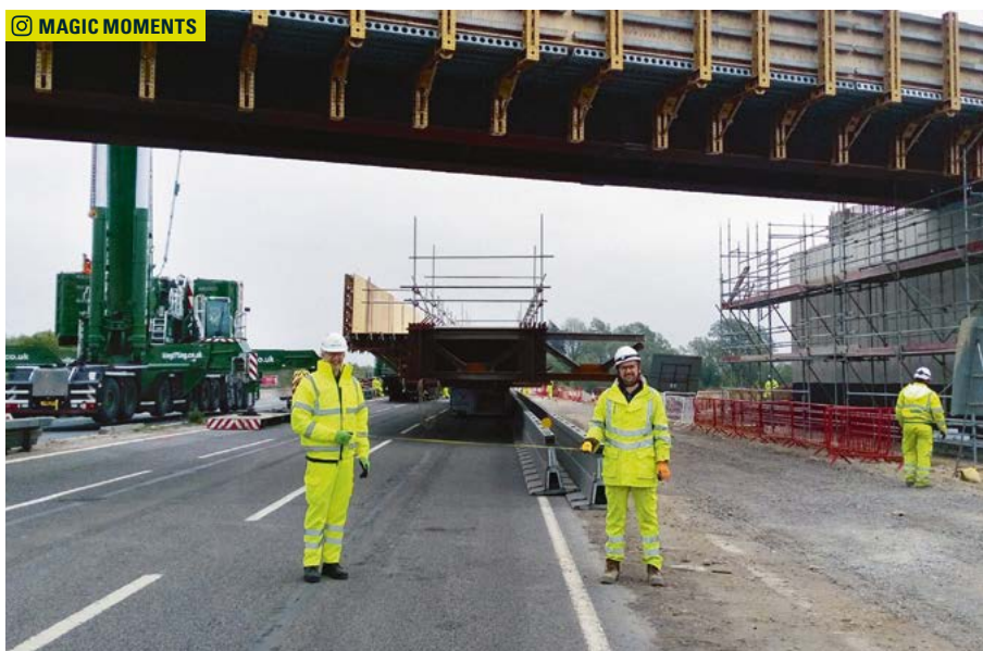
UK: The installation of a new bridge at Marsh Lane on the M4, Highways England. Photo credit: Leo Quinn
