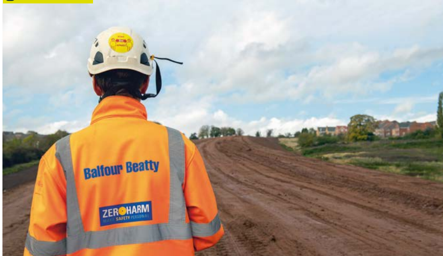
UK: Gedling Access Road, Nottinghamshire County Council. Photo credit: Paul Stephenson
