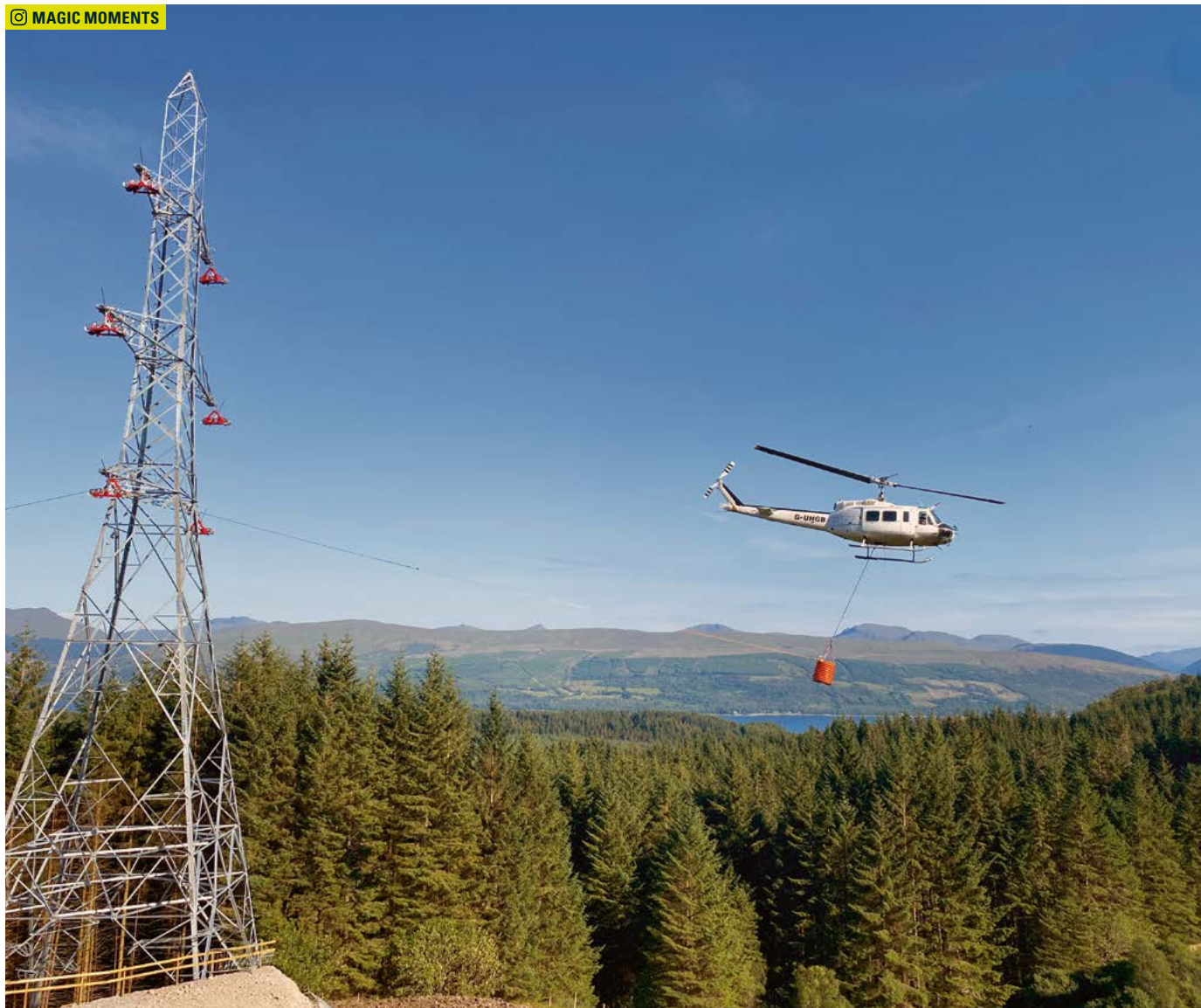
UK: Inveraray to Crossaig project, Scottish Hydro Electric Transmission (SSEN). Photo credit: Adrian Smith
