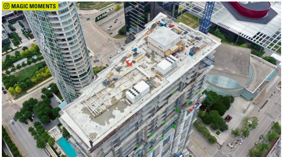
US: The Atelier residential tower, Zom Living. Photo credit: Cameron Wahl
