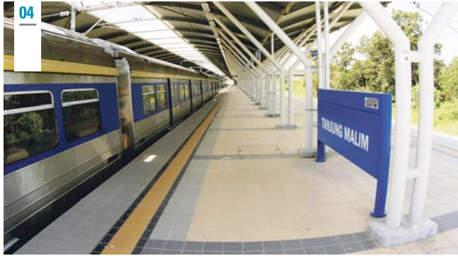
04 Rawang-Ipoh line, Malaysia – Balfour Beatty Rail International
