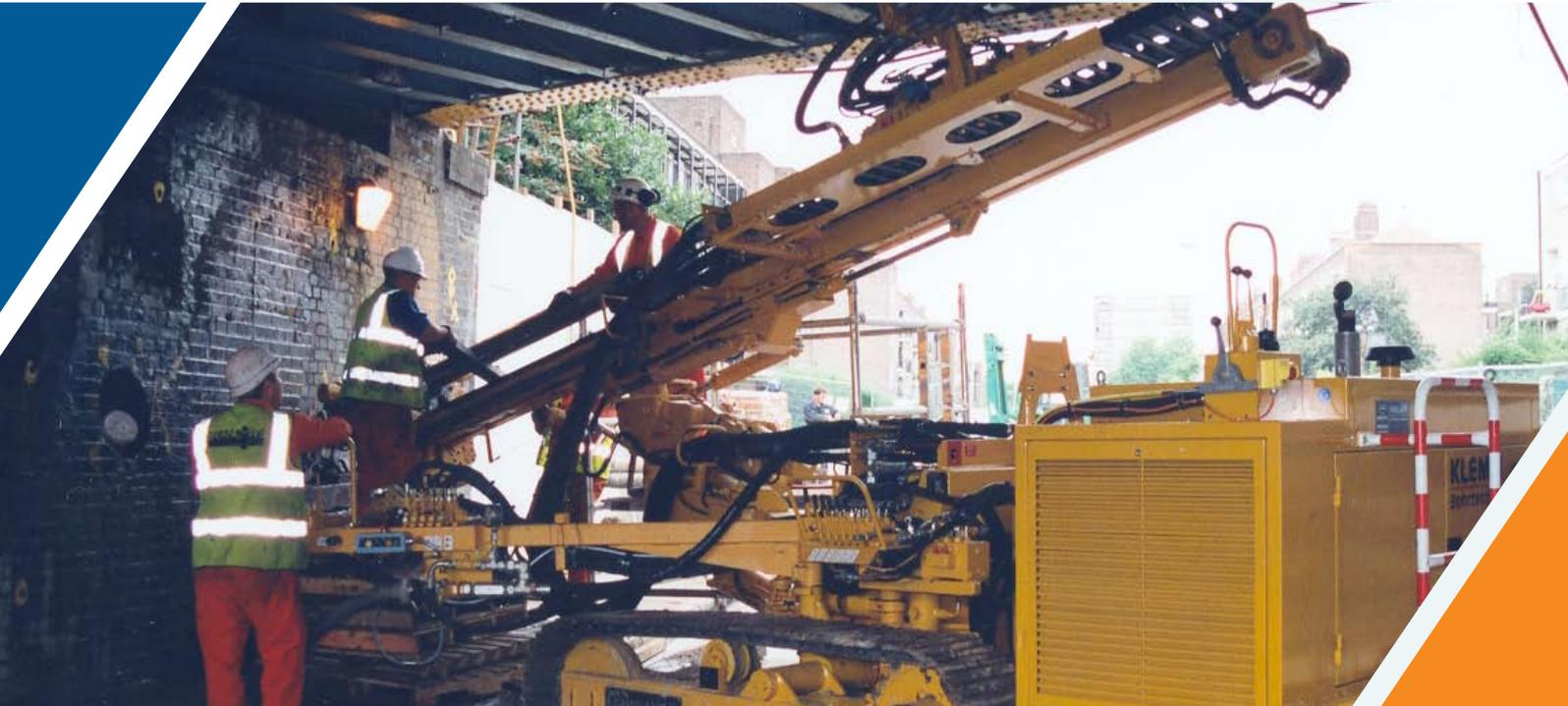
Ground Anchorages are used for a variety of applications and take a number of forms with uses for both temporary and permanent works. Simplistically they are anchorages into the ground which can be either passive or active in type.
