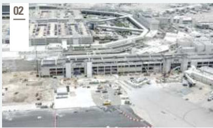
02 Miami International Airport – Heery International
