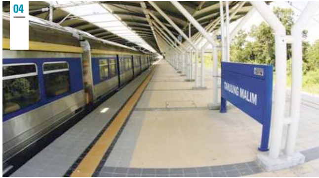
04 Rawang-Ipoh line, Malaysia – Balfour Beatty Rail International
