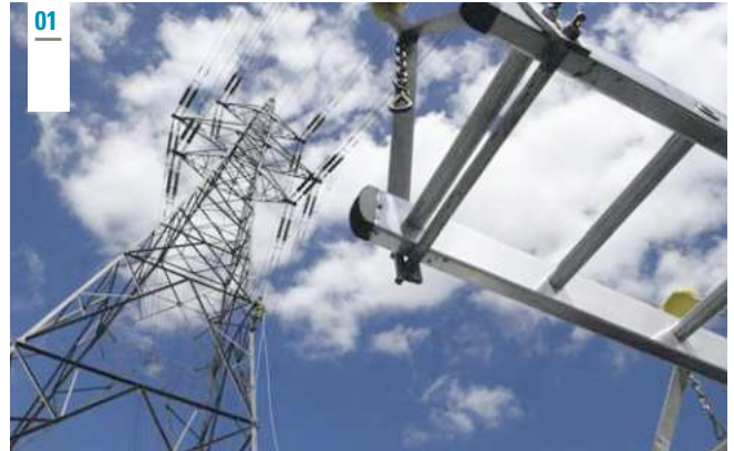
01 UK transmission system upgrade – Balfour Beatty Utility Solutions
