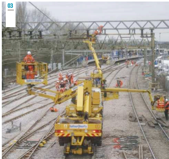
03 Network Rail track renewals – Balfour Beatty Rail Services
