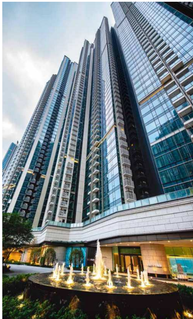
LEFT Lohas Park Package 9, development of three 54-56 storey residential towers for Wheelock and Company Limited, Hong Kong.
