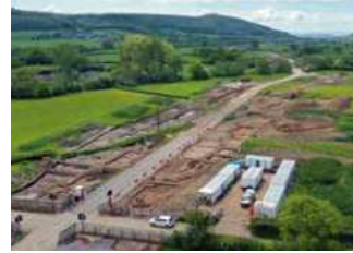
UK: Hinkley Connection Project, National Grid
